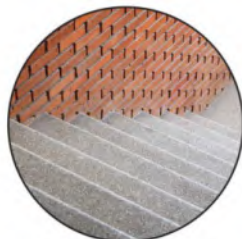
EXPOSED AGGREGATE STAIRS AND ADJOINING BRICK WALLS
