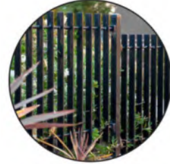
BLACK METAL SLAT FENCING. ROTATE BLADES TO PROVIDE ADDITIONAL SCREENING WHERE APPROPRIATE
